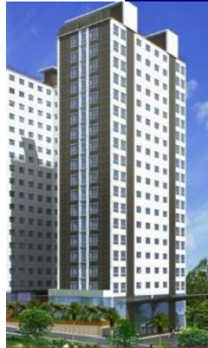
Pinewood Jatinangor Apartment - Bandung
