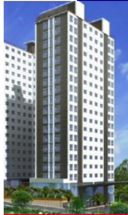
Pinewood Jatinangor Apartment - Bandung
