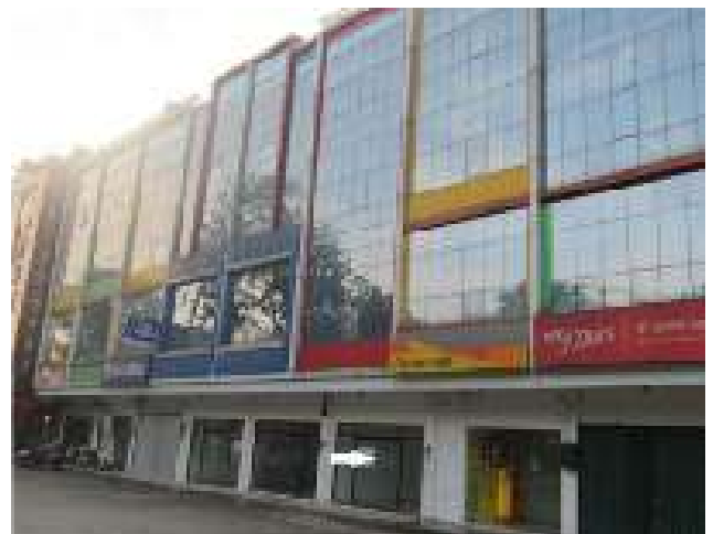
Ketapang Business Center - Gajah Mada Shop Houses - Jakarta
