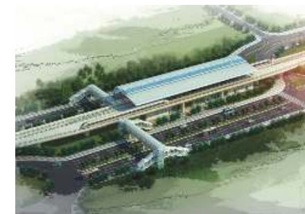
Guangzhou Metro 6 line, Guangdong, China
