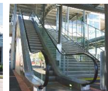
Mt Druitt Railway Station, Australia
