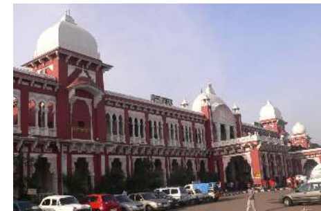
Chennai train station, India
