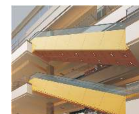
Ti-Aluminum plate LED spot lighting
