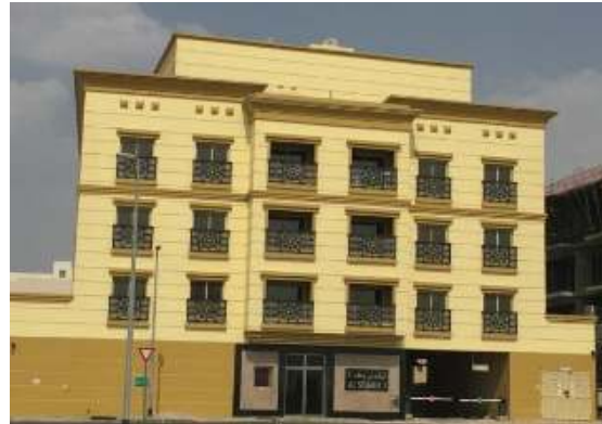
Al SHARIF BLDG, Dubai, UAE.
