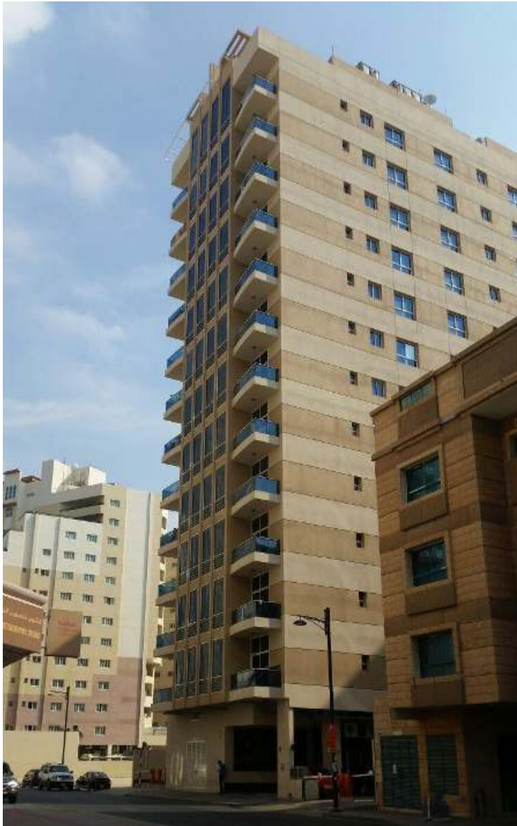
Bin Shafar Tower, Dubai , UAE.
