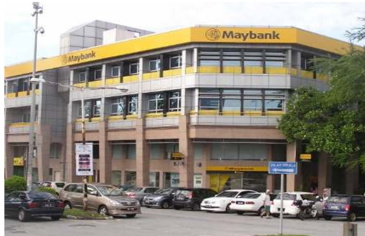
Maybank Damansara Utama, Malaysia.
