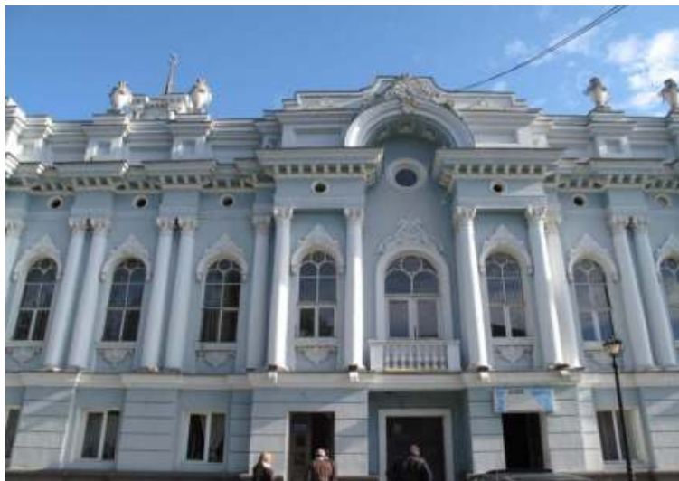
Real Invest Office Building, Georgia.
