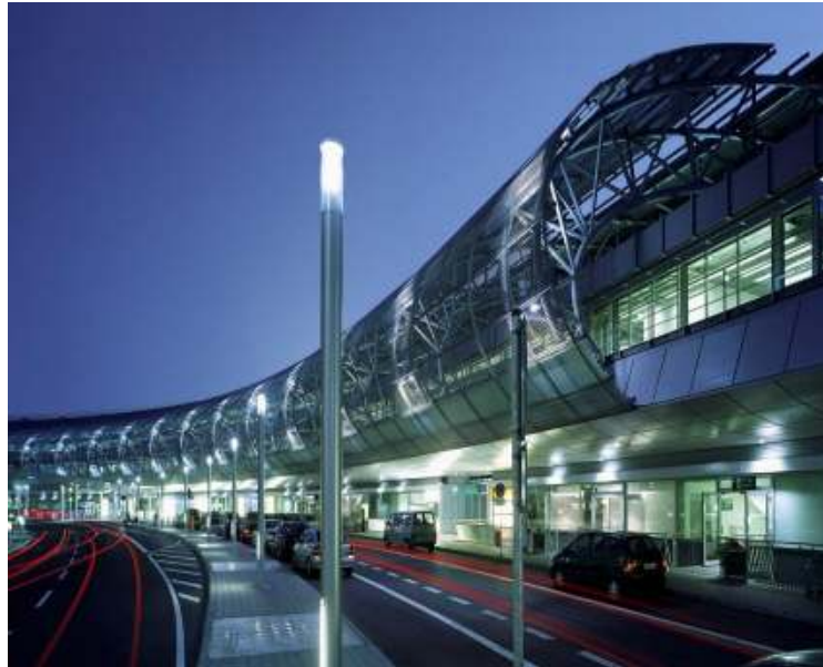
Airport Dusseldorf, Germany.
