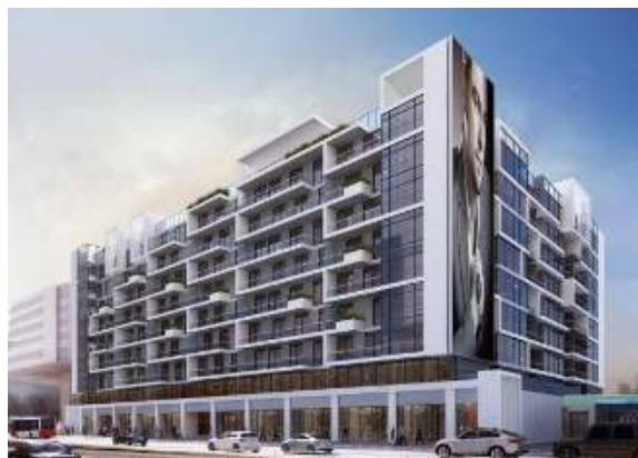
Al Shamsi Bldg, Dubai , UAE.
