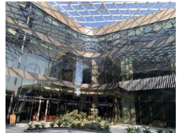
AVENUE Mall, UAE.
