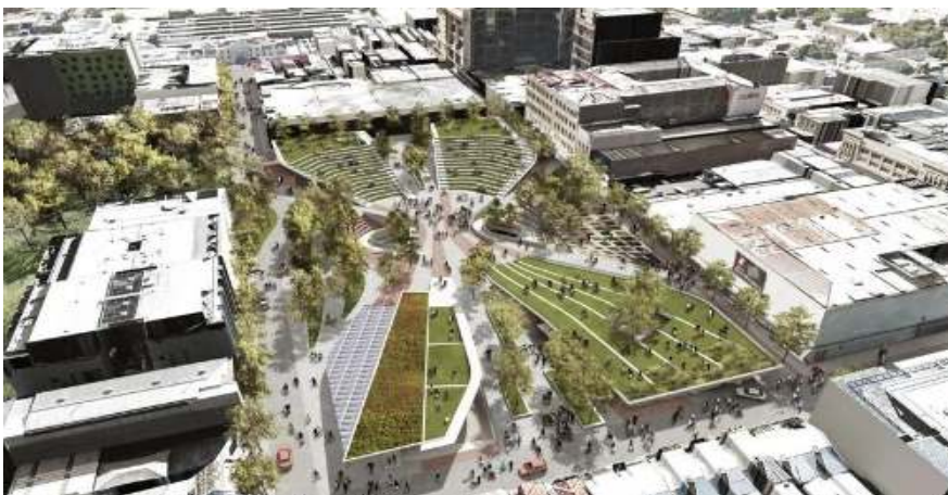
Cato Street Car Park, Australia.
